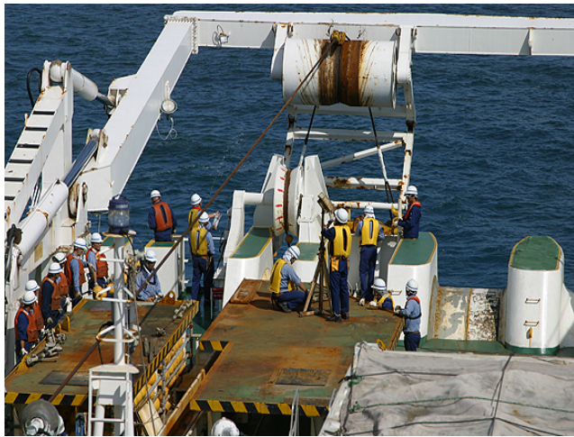
Laying down of cable/pipeline in the ocean bed
