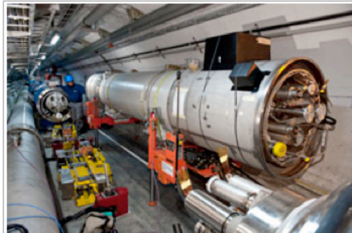
A quadrupole magnet in the LHC tunnel
