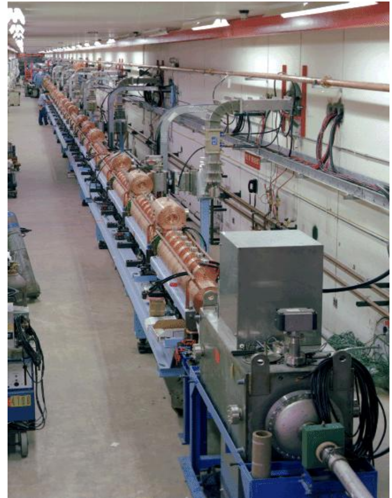
A portion of Fermilab's linear accelerator
