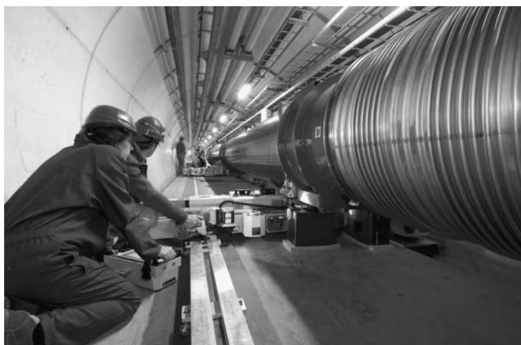
Figure 5. The first superconducting magnet for the LHC is carefully installed in the tunnel in March 2005 (photograph copyright of CERN).
