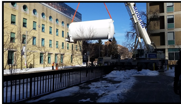
The old tank being taken away
