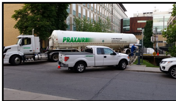
The filling of the new tank
