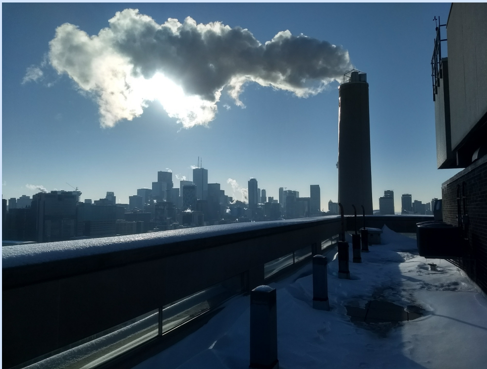
MP Balcony (Credit: Orfeo Colebatch)
