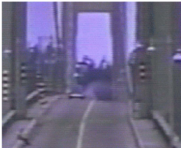
Fig. 3. Frame from the film taken by Elliot et al. (Ref. 8) of the bridge collapse. In the frame the wind moves from left to right. To the right of the car is a large vortex outlined by the cement dust from a section of the roadway that was apparently disintegrating. On the left sits Professor Farquarson. This frame is a blowup of a small section of the 8 mm film. Due to the eye's motion tracking ability, the behavior of the vortex is much clearer in the film. The roadway is almost level in its counterclockwise rotation and the low pressure vortex is thus feeding energy into the bridge motion. Copyright by The Camera Shop. Used with permission.
